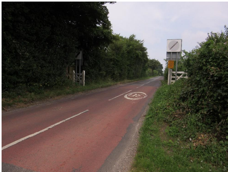
Photograph 3: Gateway signs from the rear showing how the road marking are worn and the signs hidden by the hedges.
