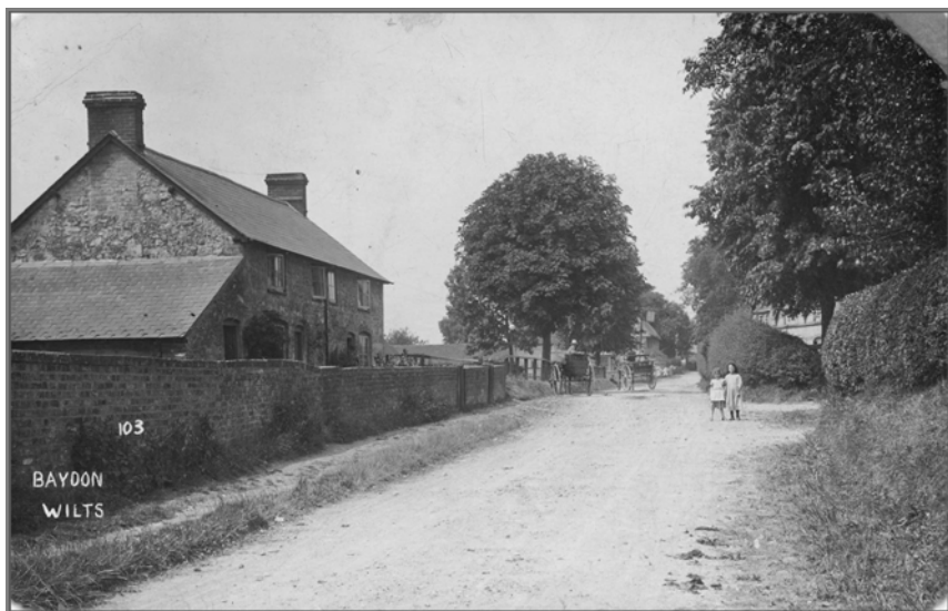
Ermin Street. Looking towards Swindon with the pub on the left beyond the carts
