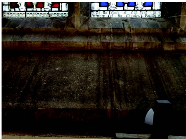
Figure 5.8 gable wall and east window cill as of 5 th April 2019 - Signs of movement in stone cill; some recent some historic.
