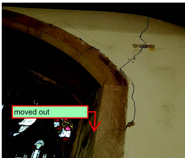
Figure 5.6 gable wall and east window as of 8 th August 2019 - Signs of new movement and in particular stone rotation.
