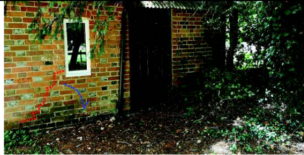
Fig 8.2 – signs of foundation movement on building next to church
