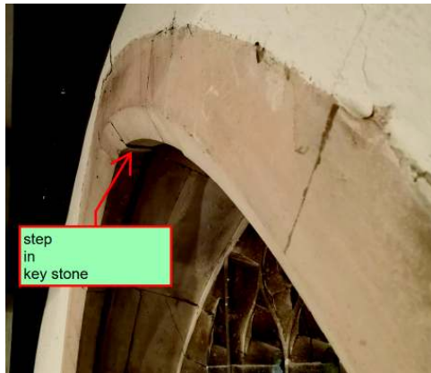
Figure5.7 gable wall and east window as of 8 th August 2019 - Signs of new movement and in particularly stone step.
