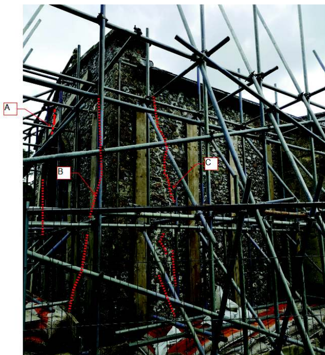
Figure 6.1 view of the North east corner with marked areas of the significant cracks in the flint work.
