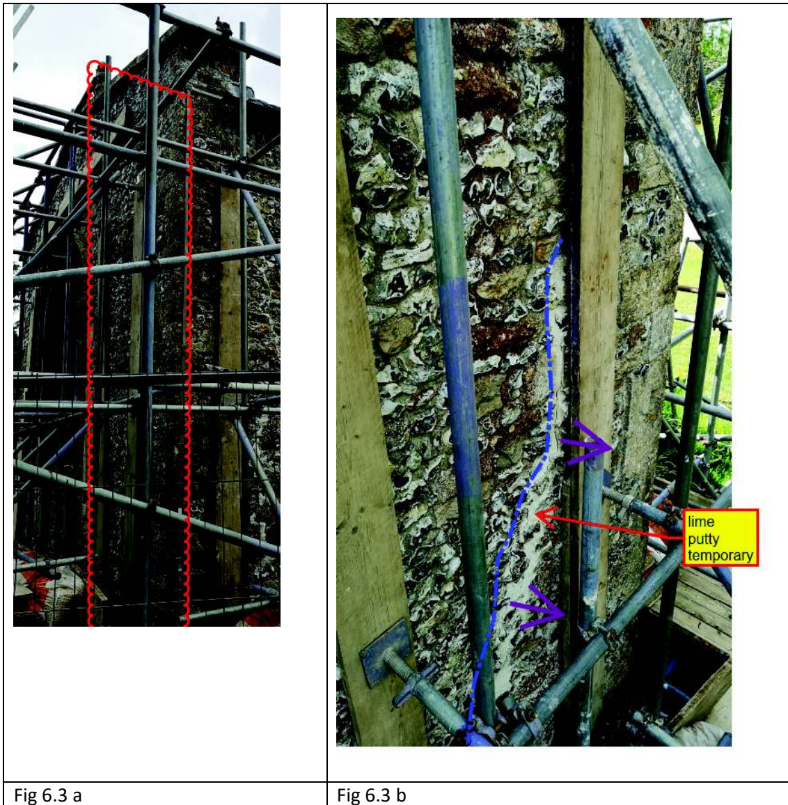
Figure 6.3 – North East corner east wall gable - crack widths vary from 2 to 10 mm. Loose failed mortar opened up cracks to suggest larger crack widths.
