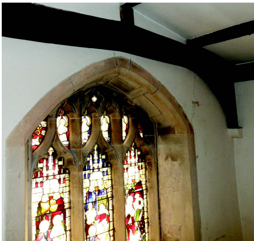
Figure 5.5 gable wall and east window as of 5 th April 2019 - Note darker pointing around the stone window frame which suggests historic repairs. There are signs of new movement and in particular the key stone at the top of the window.
