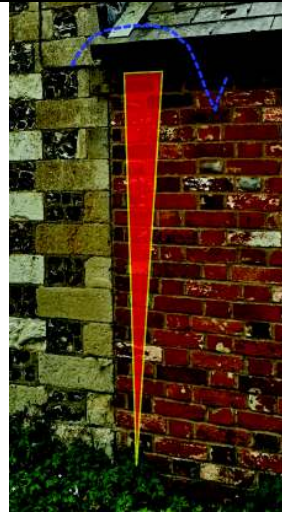
Fig 8.1 – signs of foundation movement on building next to church
