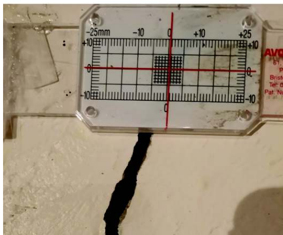
Figure 5.3 internal cracks as of 8 th August movement noted approx. 0.8mm opening – at the east gable wall.
