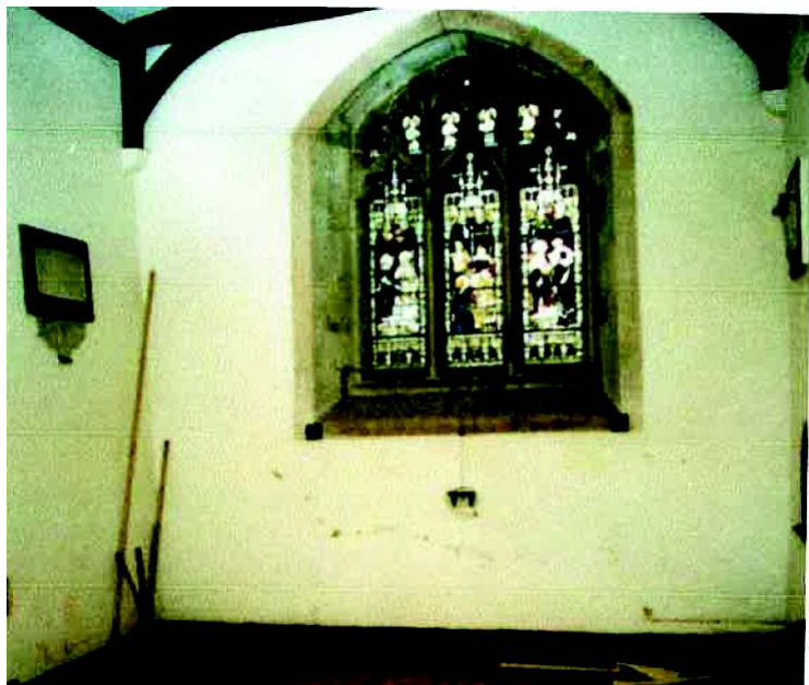
Figure 4.1- earliest photo known from 1991 when the underfloor heating was installed to the chancel area and no record or sight of the in the photo known. From the photo repairs to the mortar in the stone work over the east window key stone might be made out but this is not proven.
