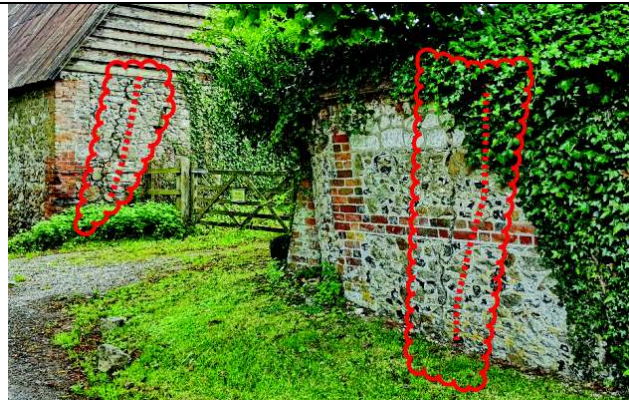
Fig 8.4 – signs of foundation movement and thermal movements on clunch and flint walls near to the church
