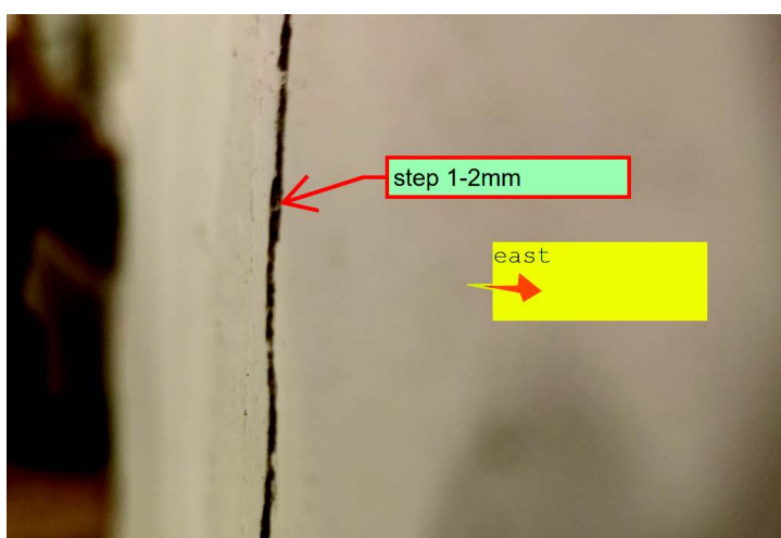
Figure 5.4 internal cracks as of 8 th August movement noted approx. 0.5mm step rather than increase in width – at the north wall.
